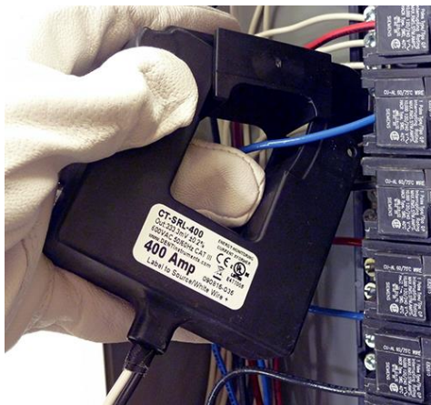
Photo 2: Install CT Around Conductor.
